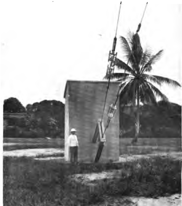
FIG. 136.—Aerial anchorage of Quenched-Spark wireless station at Jesselton (British North Borneo).
